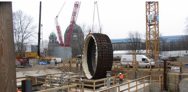
■ Starting ring for the HDS TBM
