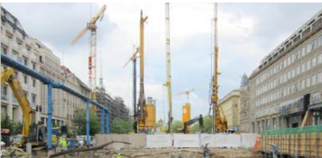
■ Cut and cover excavation of a station
