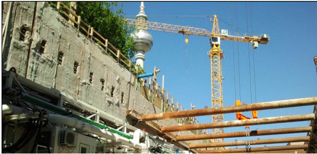
■ Starting shaft for TBM
